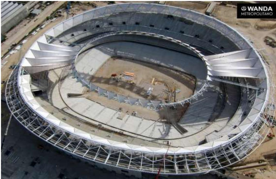
The roof is one of the most significant elements, and largely responsible of the stadium's image. It's also the element that protects spectators from the inclement weather and standardizes the building, as it merges the original part from la Peineta (the previous stadium) with the enlargement of the new stadium. It has a height of 45 and 57 meters in relation to the pitch.
